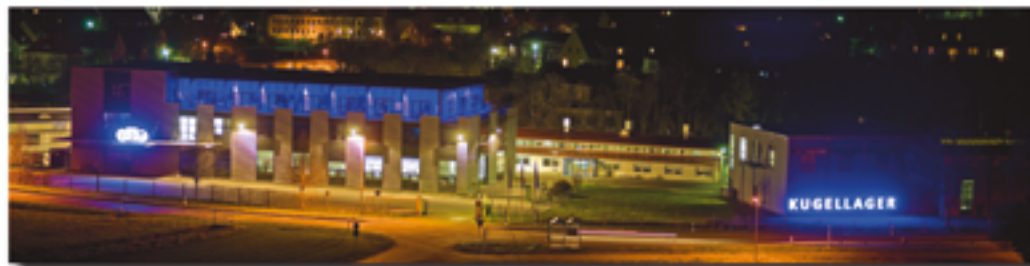
Administration and production facilities Rimpar
